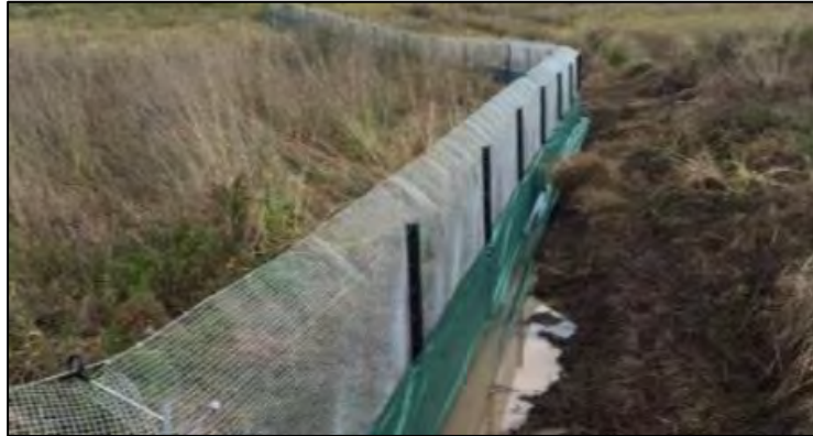
Plate 10. Example of suitable frog exclusion fencing (fence posts must be on the outside and not within the Habitat Corridor)
