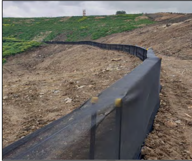
Plate 9. Example of suitable frog exclusion fencing
